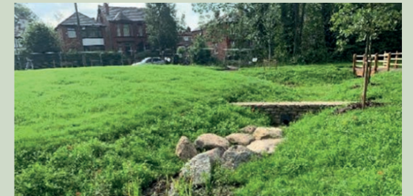
Figure 14 Main swale and check dam flow control feature, showing wetland planting and boulders placed to remove energy from circulating flows.
