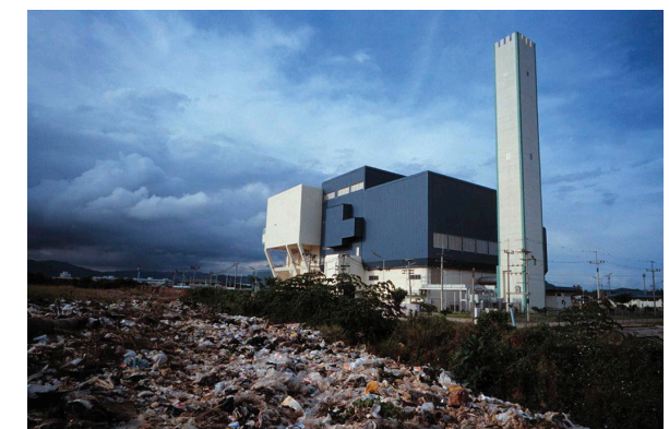
Energy from waste plant. Image source: Construction News
