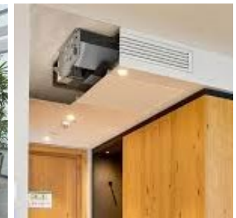
Ceiling mounted fan coil unit
