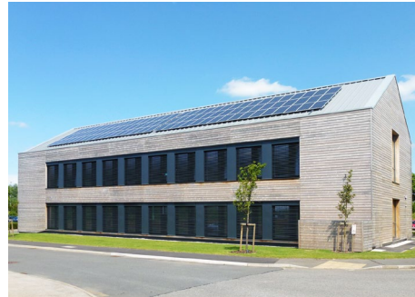
Image source: CPMG Architects
