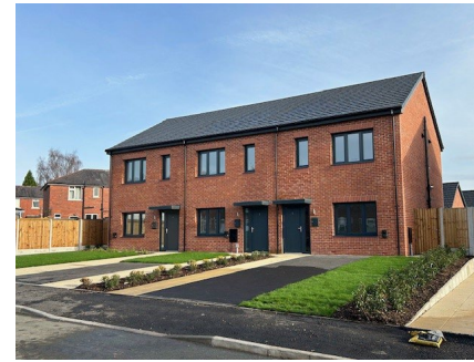
Image source: RP Tyson Construction
